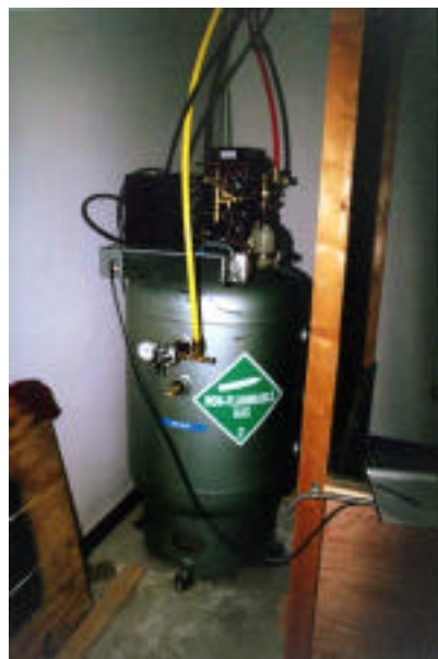
Ballast tank with compressors. Gas bag to right. Cost of equipment in room - approximately $5000.
